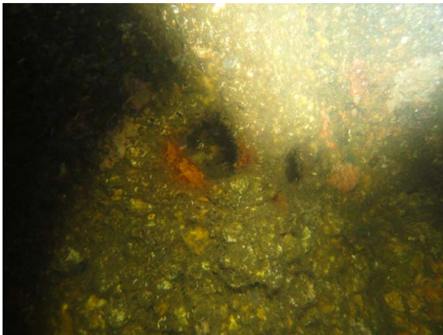
Photo 4: Typical Small Holes Through Sheet Piling Extending into Concrete Face of Caisson.
