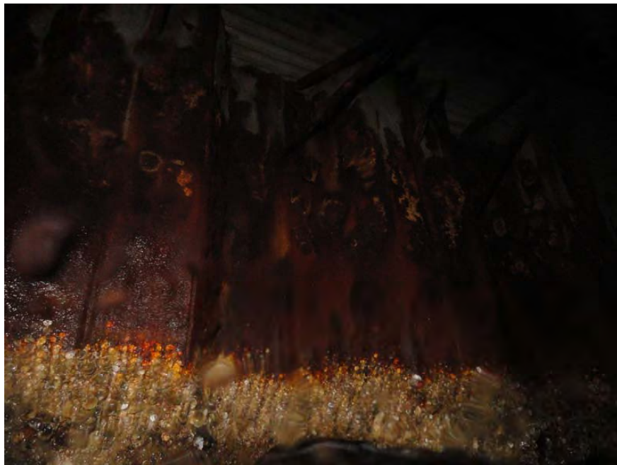
Photo 2: Typical Heavy Corrosion on Sheet Piling in the Tidal Zone.
