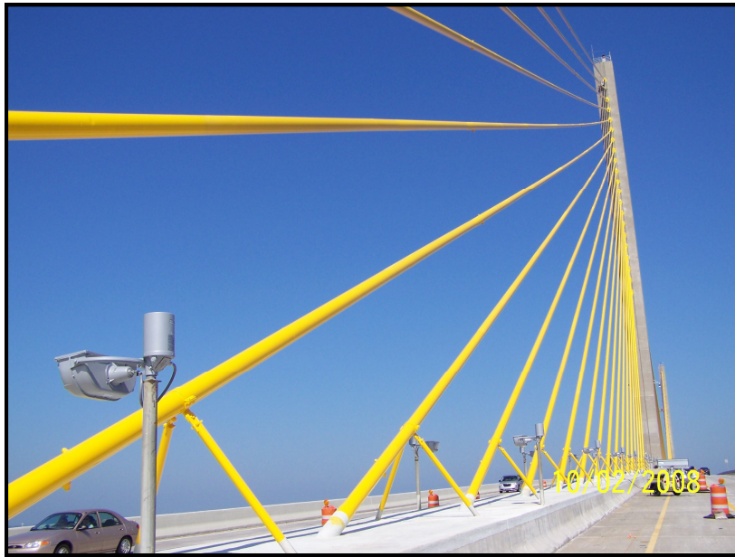
Figure 4- Completed section in October 2008 of the yellow color with the clear coat chosen by FDOT.
