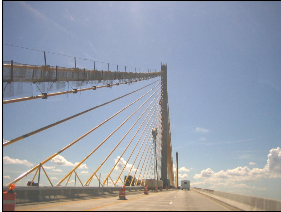
Figure 5- Rigging on Stay cables 21 & 20
