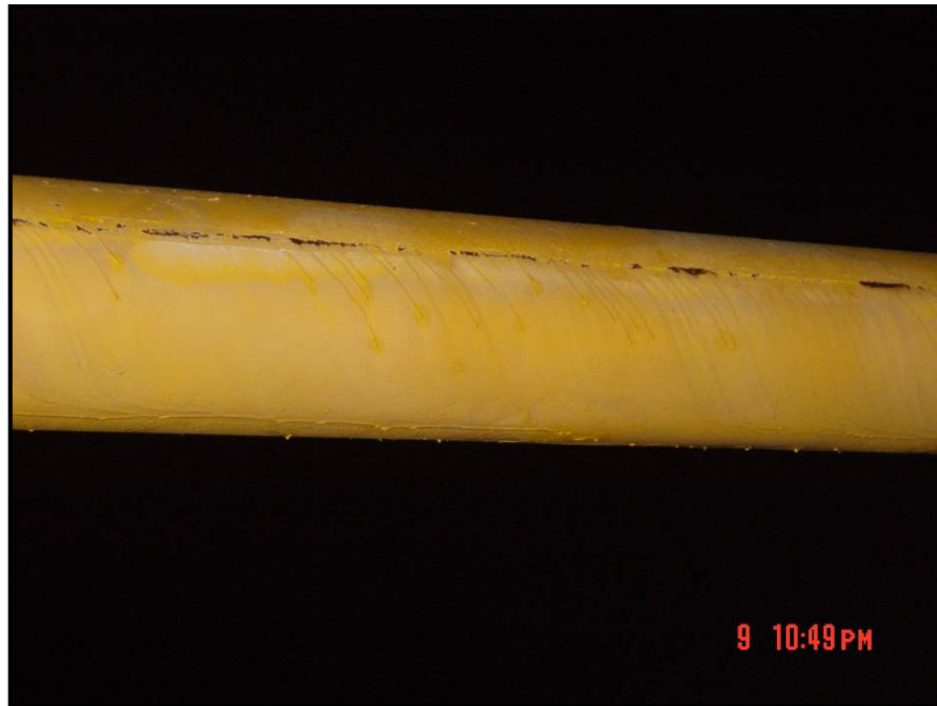
Figure 3- Corrosion typical of the condition on stays in the upper areas at project start-up.
