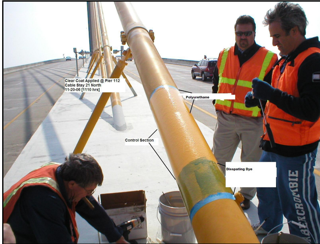
Figure 8 – Application of clear coat with dissipating dye.
