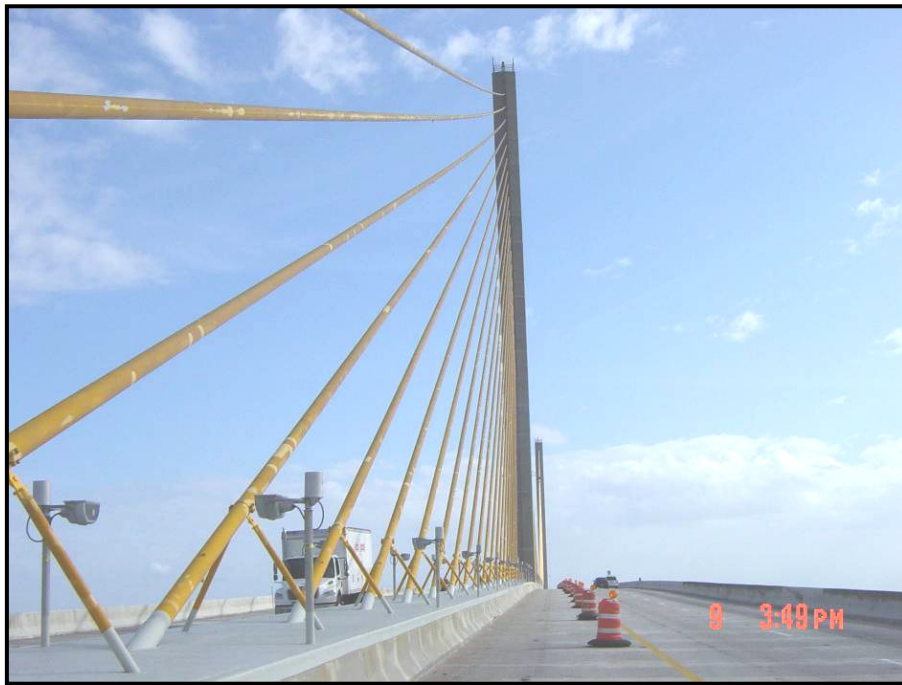
Figure 1- Sunshine Skyway pre-project typical spot coat appearance.
